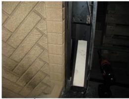
Using a <sup>3</sup>/<sub>8</sub>" wrench or a Vise-Grip type wrench, open the threaded connector and remove the cable.
