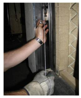
Remove the counterweight blocking rod and lower the counterweight all the way down. It will drop down several inches.
