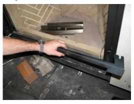
You can stop here if you only want to change the stainless steel gasket at the bottom of the guillotine frame.
